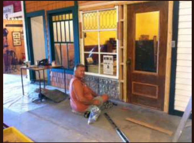
Richard Geisler applying tin siding
